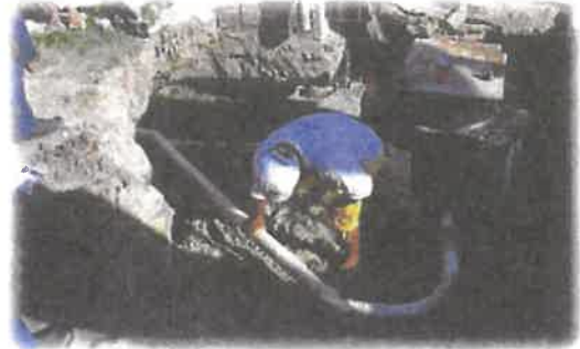
Interconnection process, of gravity and vacuum lines.
