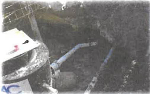
Interconnection process, of gravity and vacuum lines.
