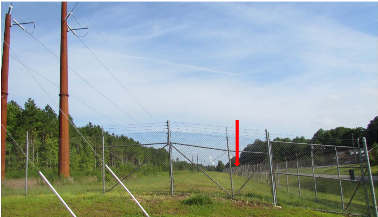
Figure 4: Proposed location of line paralleling 115kV line along Ken Trowbridge Rd. Gas line marker identified in photo.
