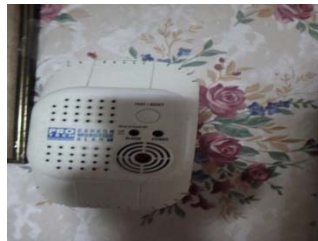
Non-Functioning CO Detector
