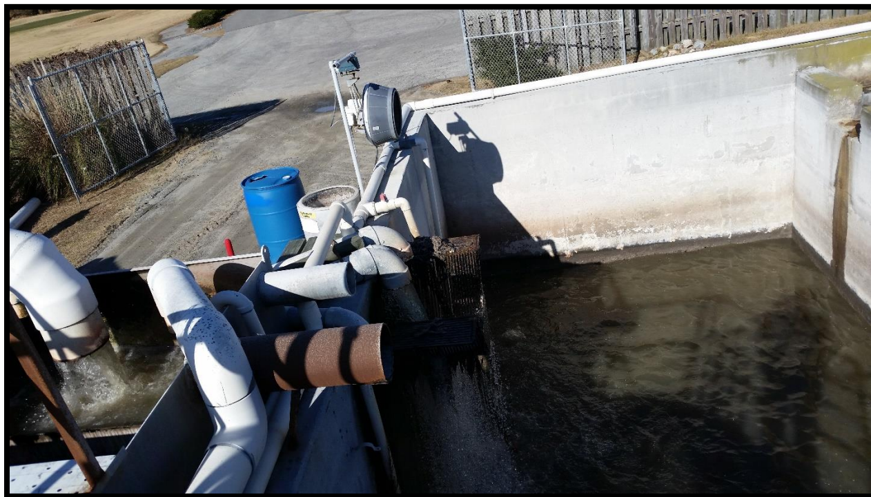
Photo 4 - Force Main from Pump Station 1 Discharging into Bar Rack, Oscillating Ecosorb® Distribution Fan Beyond
