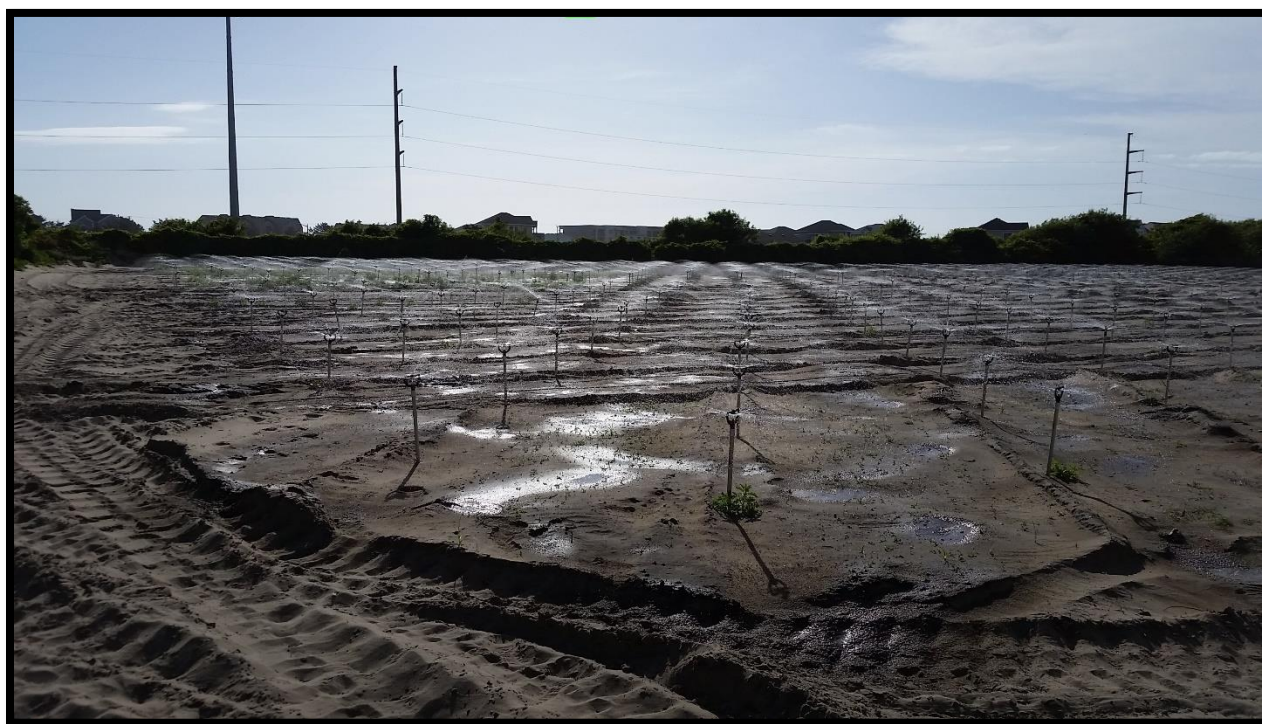
Photo 1 - High Rate Infiltration Spray Beds
