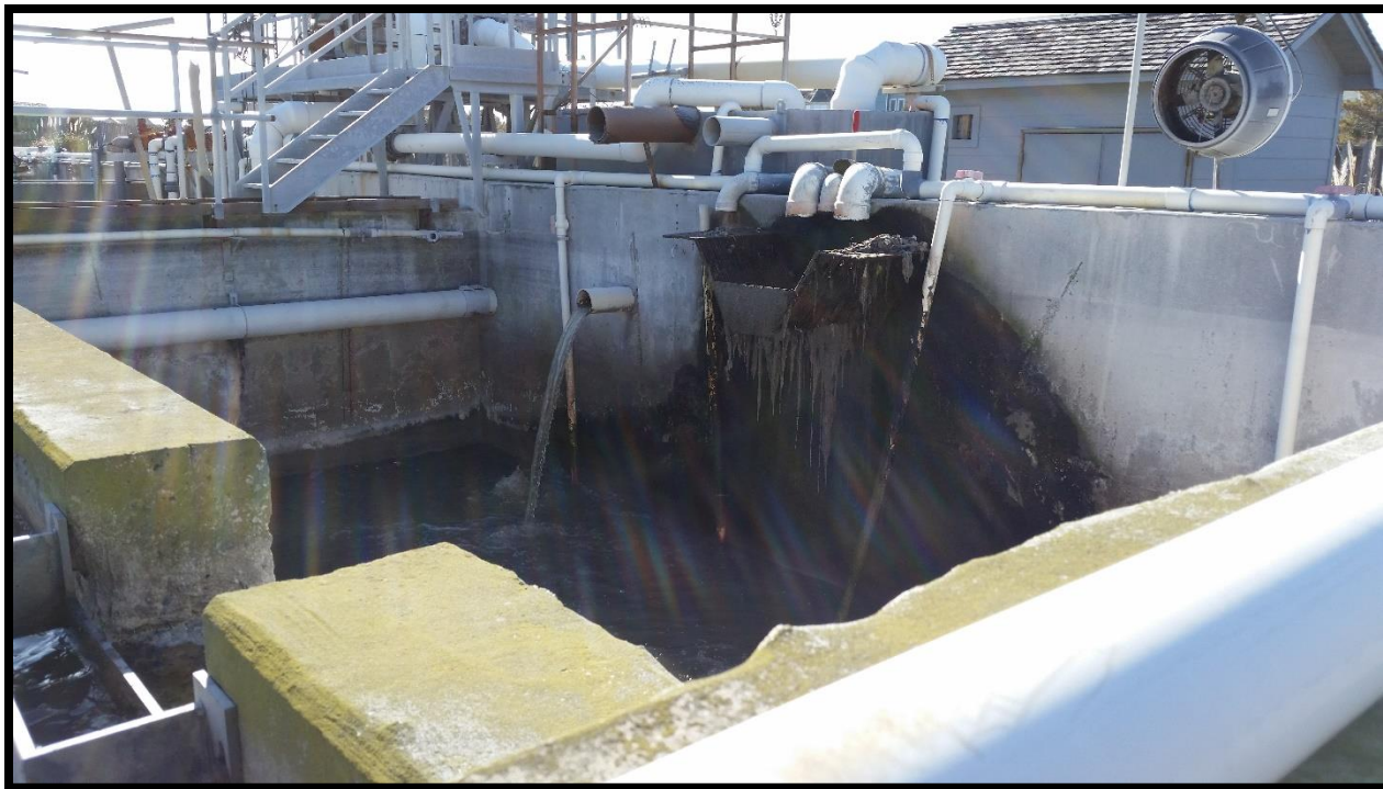
Photo 2 - Manually Cleaned Bar Rack with the Three Force Main Discharges Above and the Flow Equalization Basin Below
