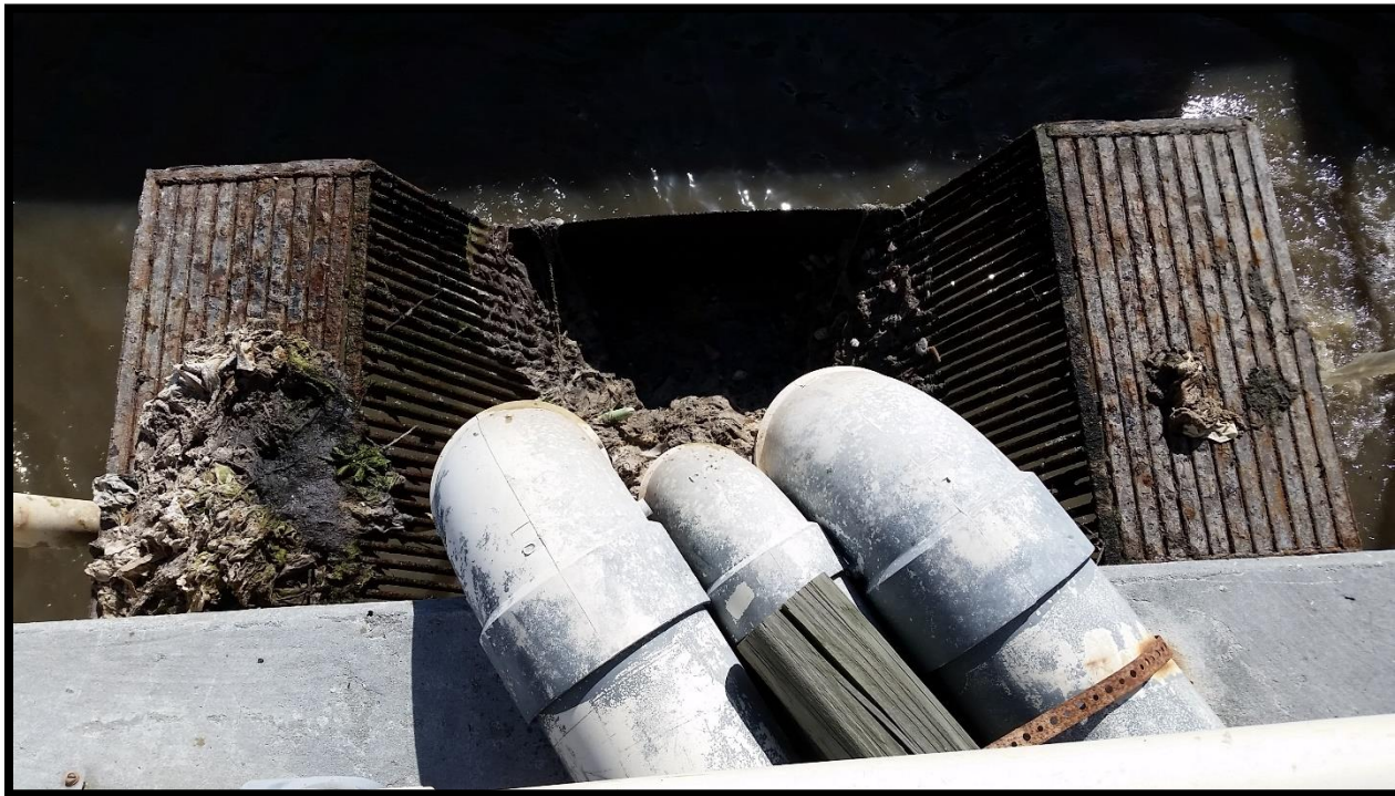
Photo 3 - Discharge Point of Three Force Mains onto Manually Cleaned Bar Rack
