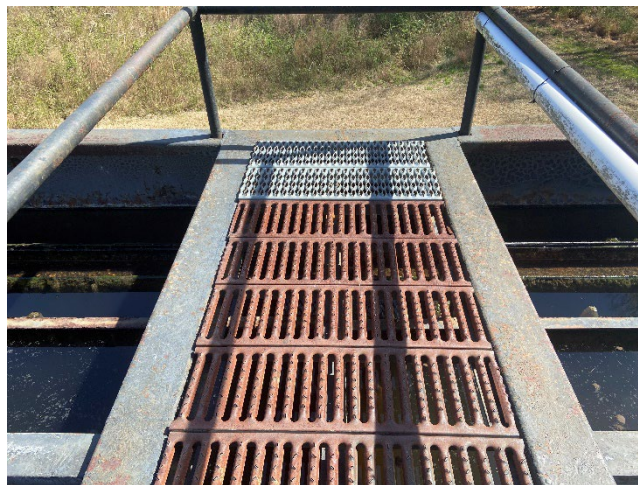
Deteriorating catwalk treads.
