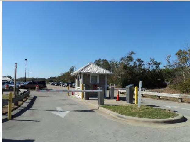
Typical Parking Attendant Station
