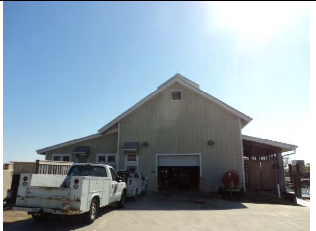
Ferry Repair Building
