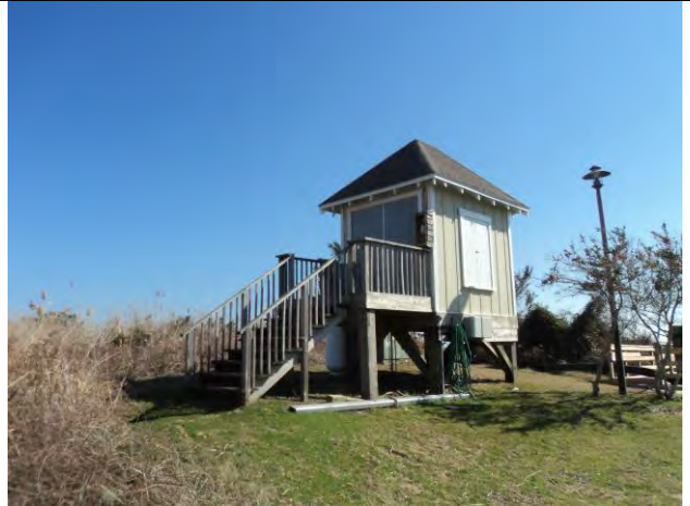
Barge Lift Mechanical Building
