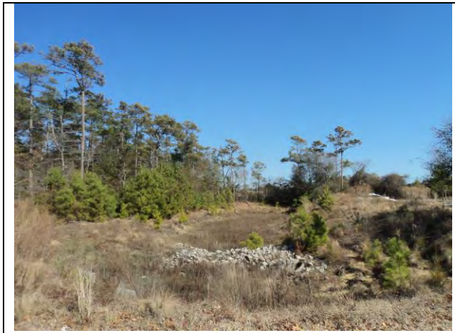
Storm Water Retention Pond
