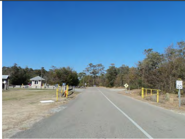
Typical Access Road
