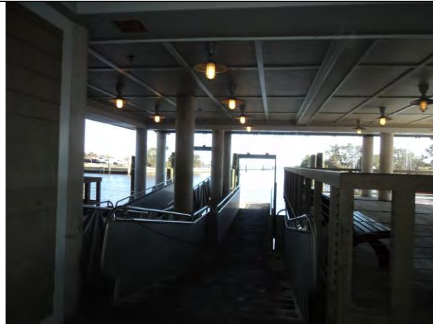
Passenger Boarding area
