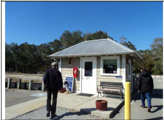
Typical Parking Attendant Station
