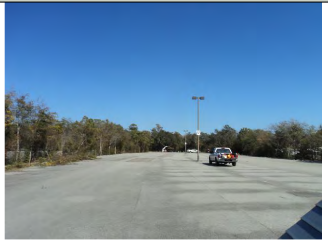
Typical Parking Area
