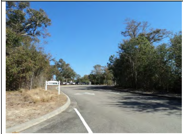
Typical Access Road
