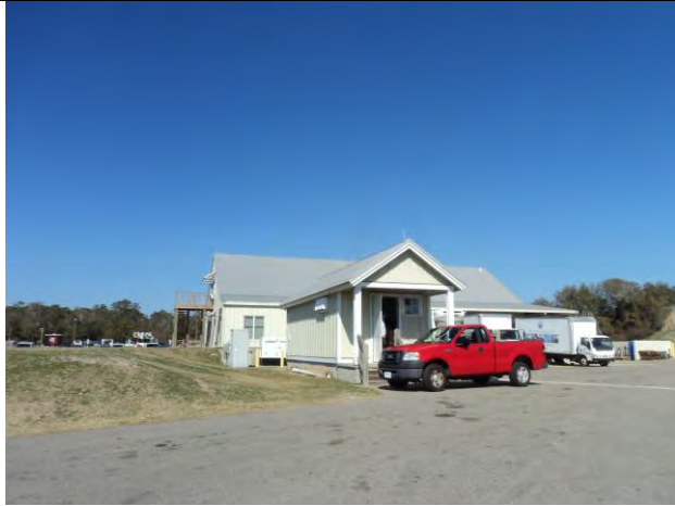
Computer Server Building
