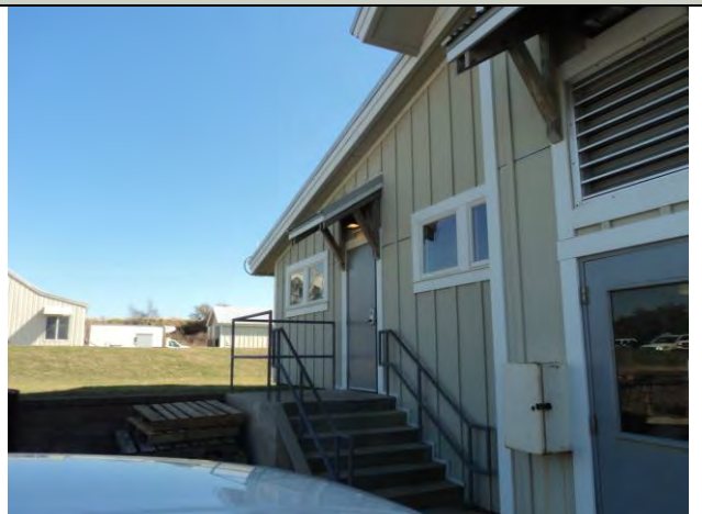
Ferry Repair Building
