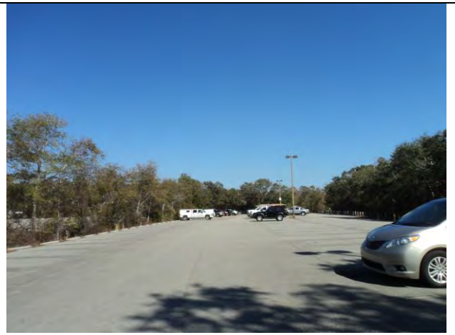
Typical Parking Area
