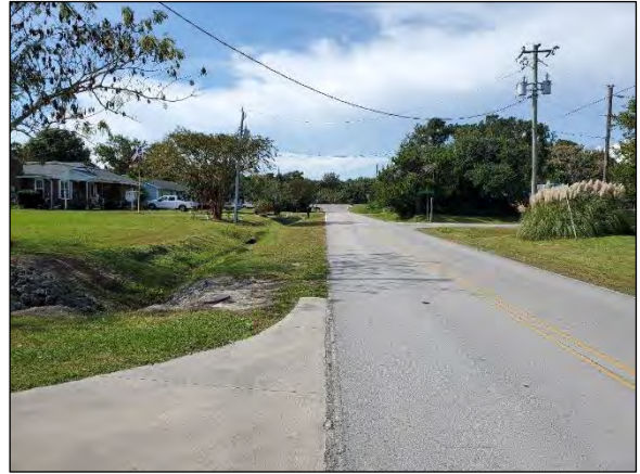
Looking northwest along Shell Landing Road, subject on left
