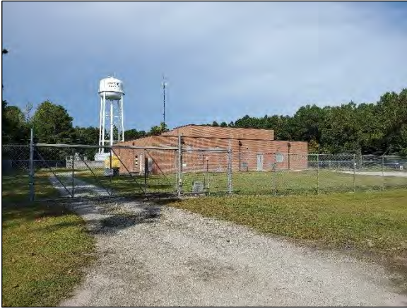
Interior view of parcel, facing northeast
