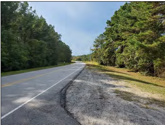
Looking west along US Hwy 101, subject on right
