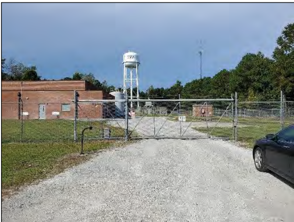
Looking north through east entrance to parcel
