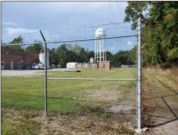
Interior view of parcel in distance, facing northwest
