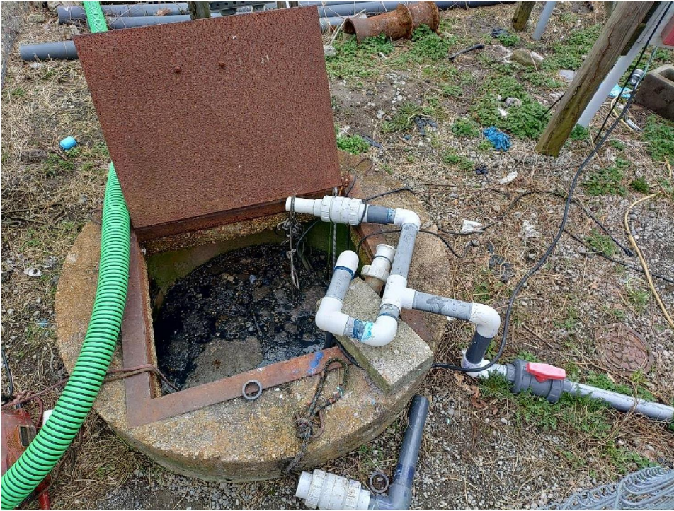
Figure 1. S. Ivon Dr. Pump Station
