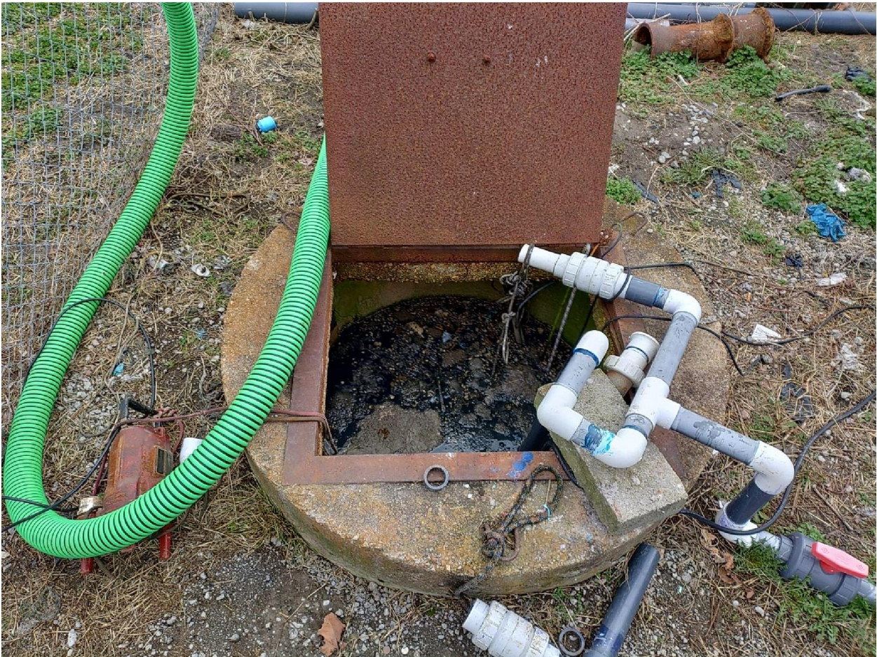
Figure 2. S. Ivon Dr. Pump Station
