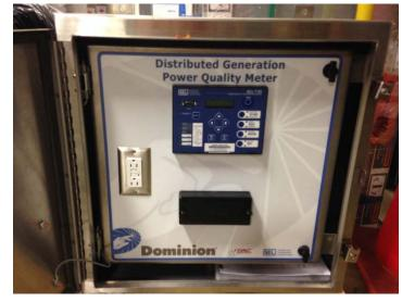
trip on various UL1741 set points (e.g. low voltage, and backfeeding the power grid) and has the ability to be remotely tripped by a Company operator. This relay configuration allows Company operators to remotely and safely isolate the micro-grid generation from the local grid when required due to line maintenance or field switching events.
