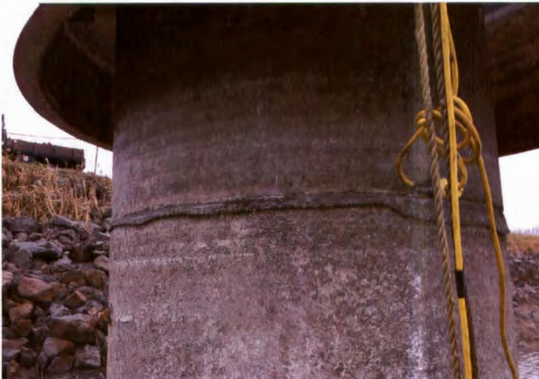
**Photograph 14.** 3/19/14 photograph of new grout on CAPE FEAR coal ash basin riser.
