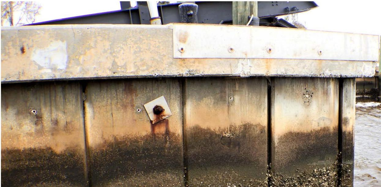
Photo taken from inlet channel showing affected concrete panels, steel tie rod with square plate washer, and steel repair plate on the concrete cap
