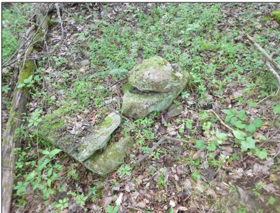
Figure 5.64. Fieldstone footer at site 31MG2261.
