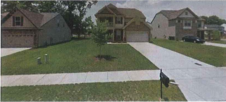
5406 Ophela Ct SW Building
