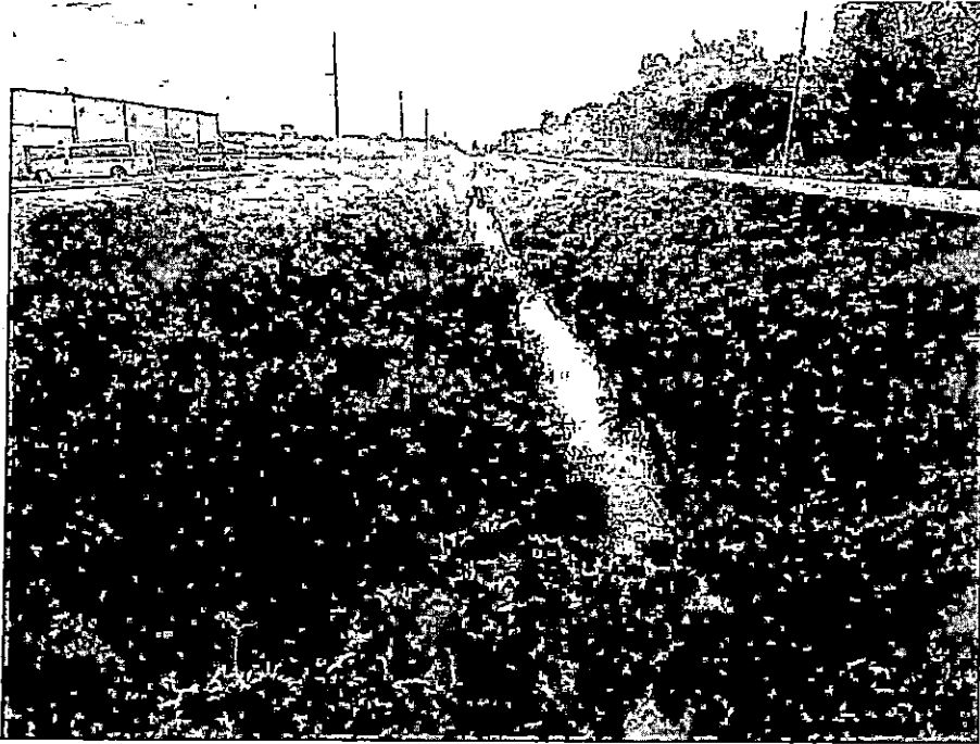
Photo 3: Looking east from intersection of Terra Ceia Road and Christian School Road at large canal that intercepts small canals. All project drainage exits to this tributary.
