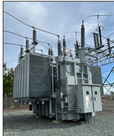
230/100kV Autotransformer
