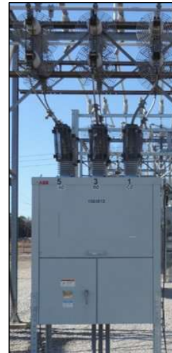
Distribution Vacuum Circuit Breaker (VCB)
