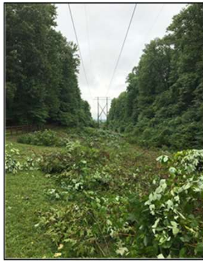
Removal of incompatible vegetation along Transmission ROW
