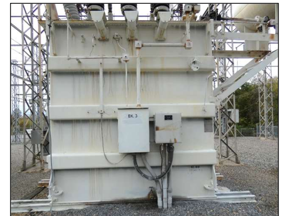
Concord Mn 100/13kV Transformer
