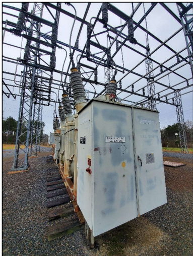
Shelby Tie 100kV Oil Circuit Breaker
