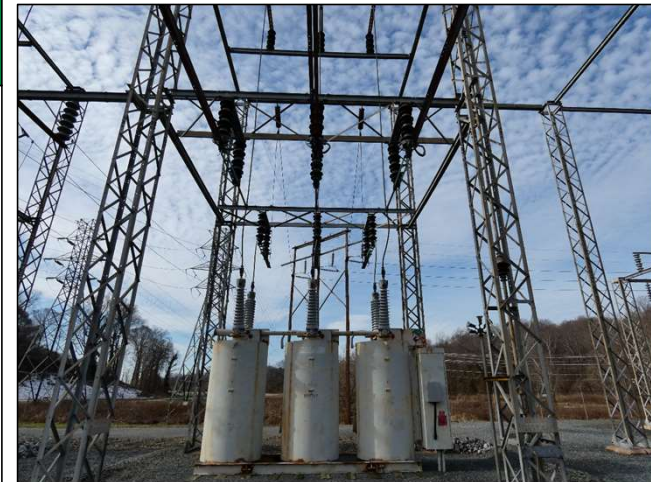
Substation Oil Breaker
