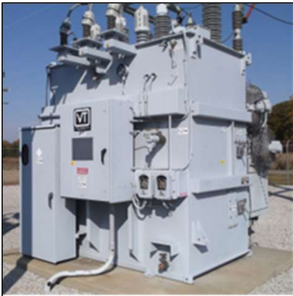
Typical T/D Transformer
