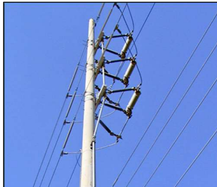
Remote operated line switch
