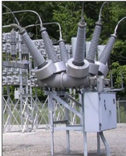
Transmission Gas Circuit Breaker (GCB)
