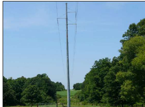
Line Rebuilt to 100kV Standard
