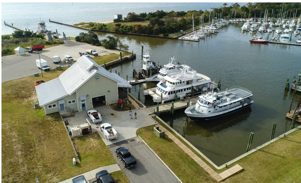
4 5 Figure 5: The Marine Maintenance Facility at Deep Point
