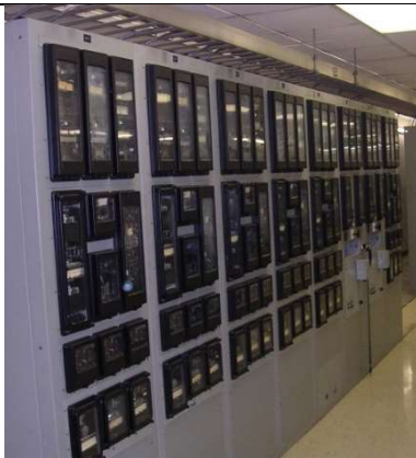
Typical electromechanical relays
