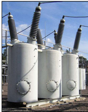
Typical Transmission Oil Circuit Breaker
