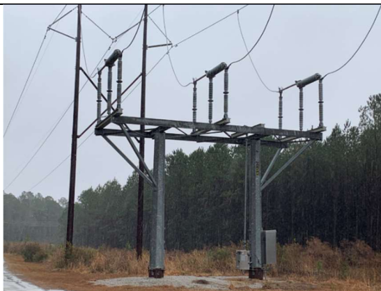
Remote-controlled switches
