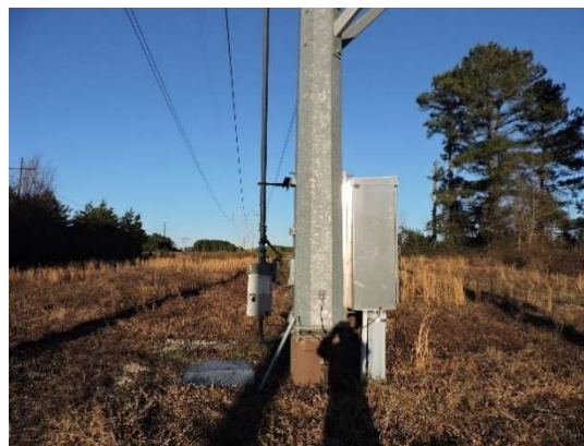
Control box for switch operations
