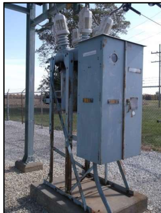
Typical Distribution Oil Circuit Breaker
