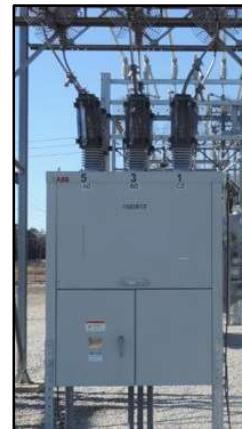
Typical Distribution Vacuum Circuit Breaker
