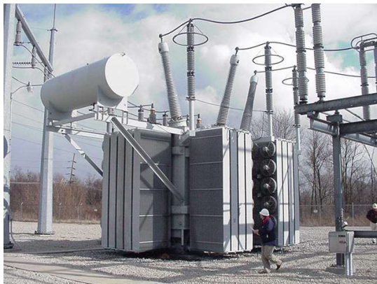
Typical transmission transformer
