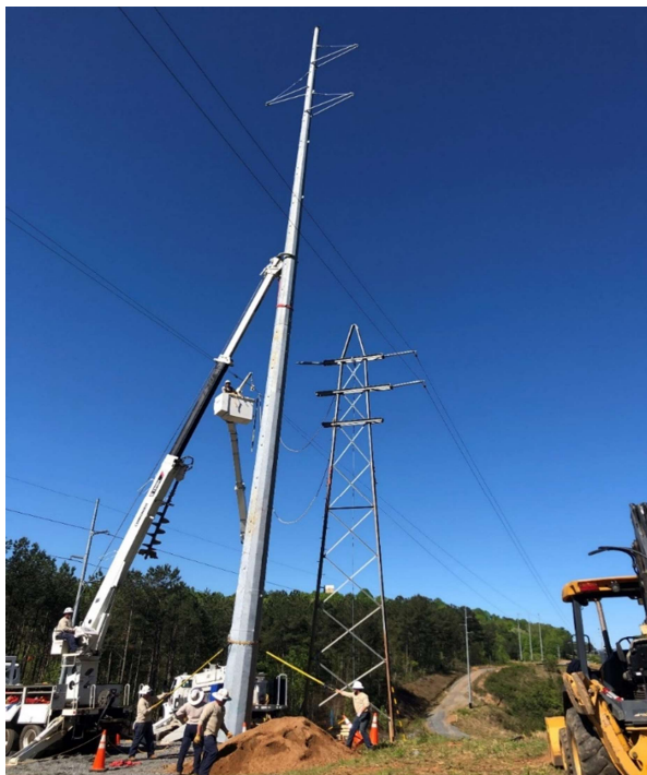
Typical 44 kV Line Being Rebuilt
