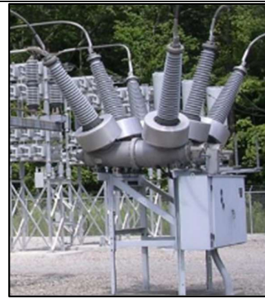
Typical Transmission Gas Circuit Breaker
