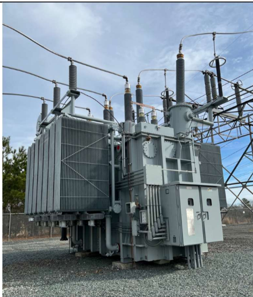
230/100-kV Autotransformer
