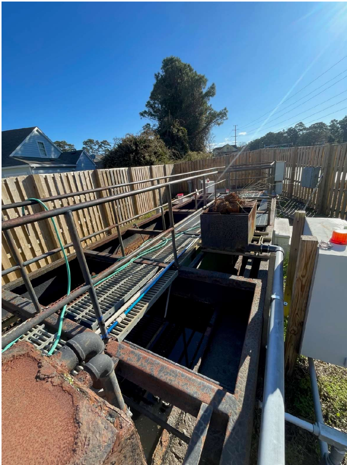
Back end of WWTP
