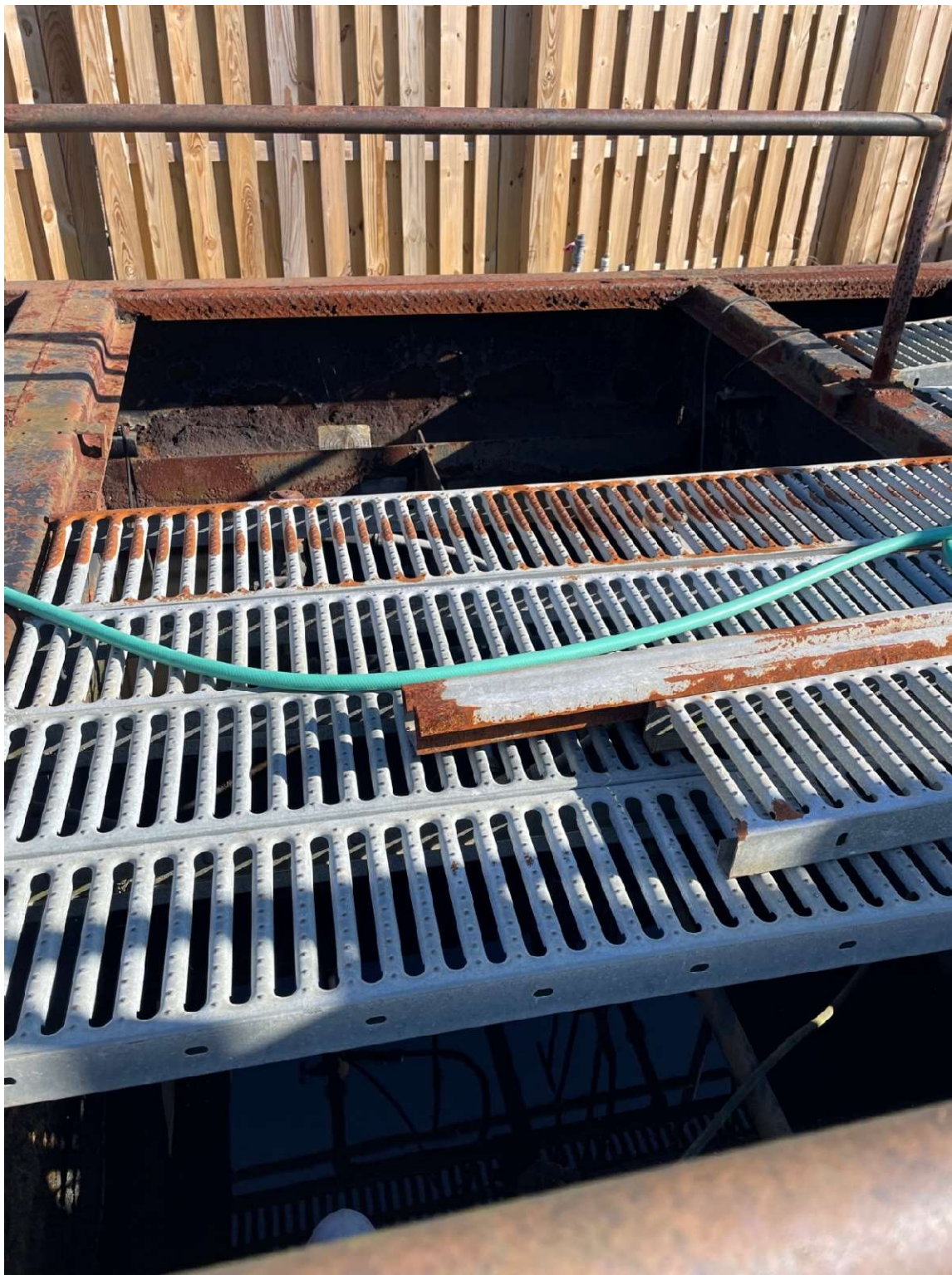
Back end of WWTP
