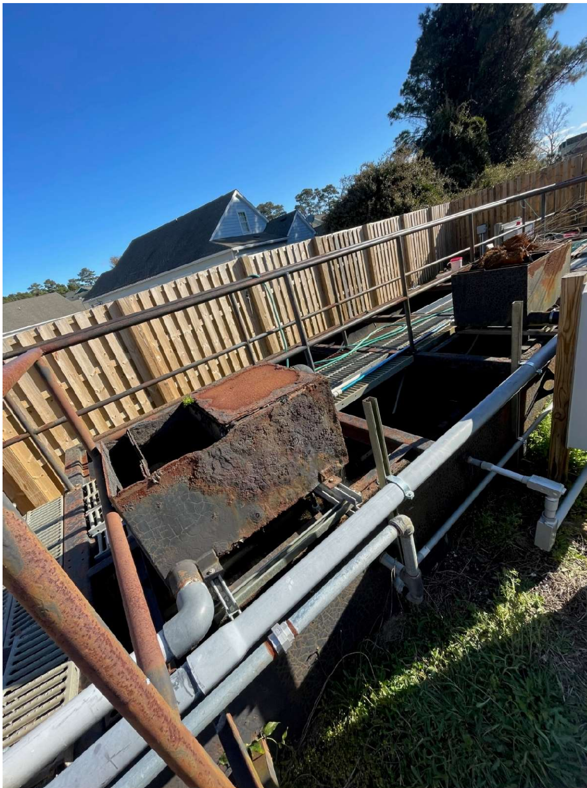
Back end of WWTP
