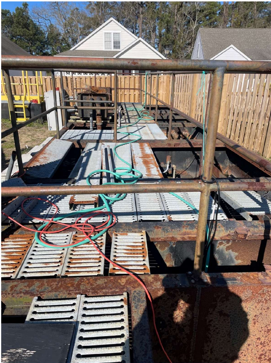
Back end of WWTP
