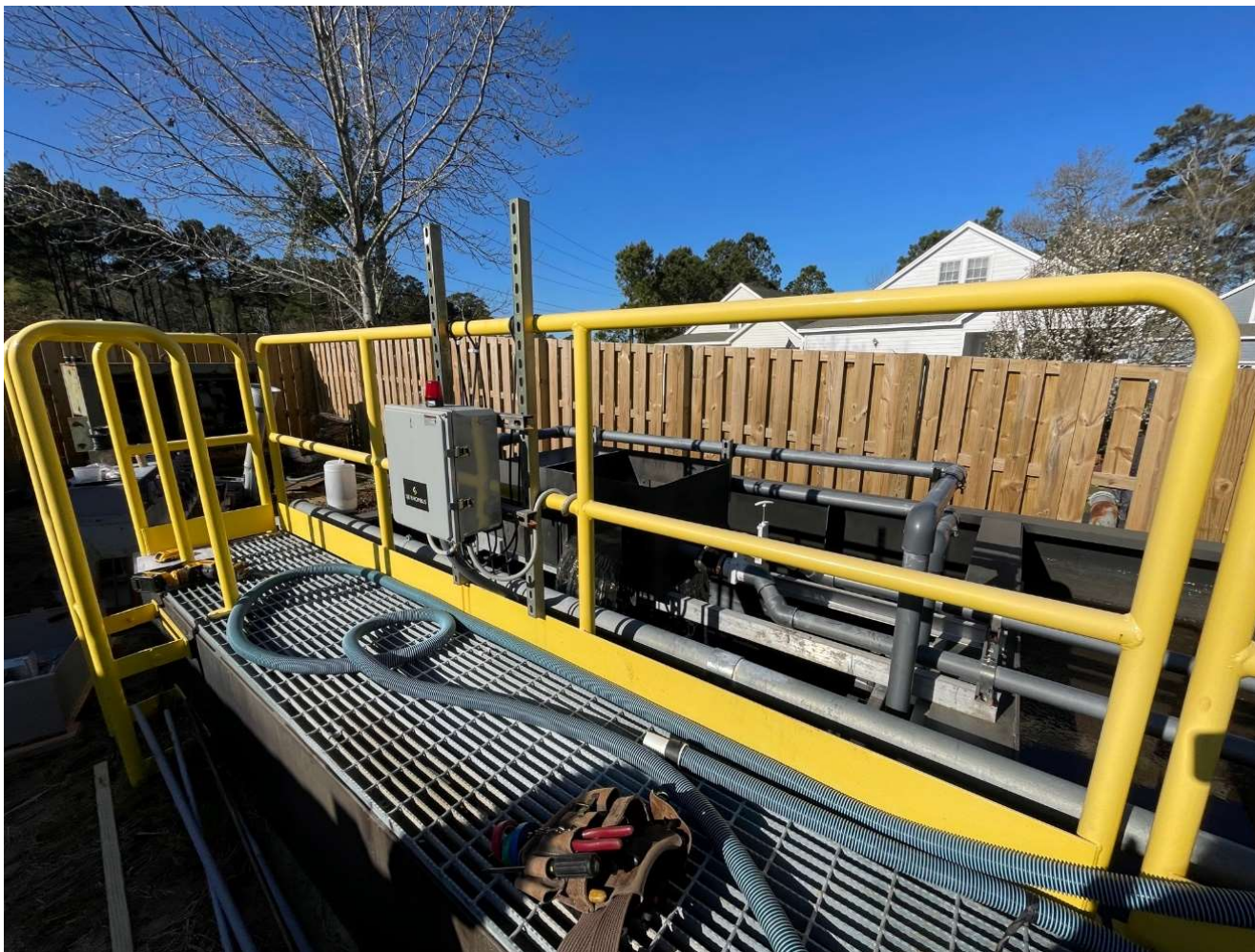
Front end of WWTP
