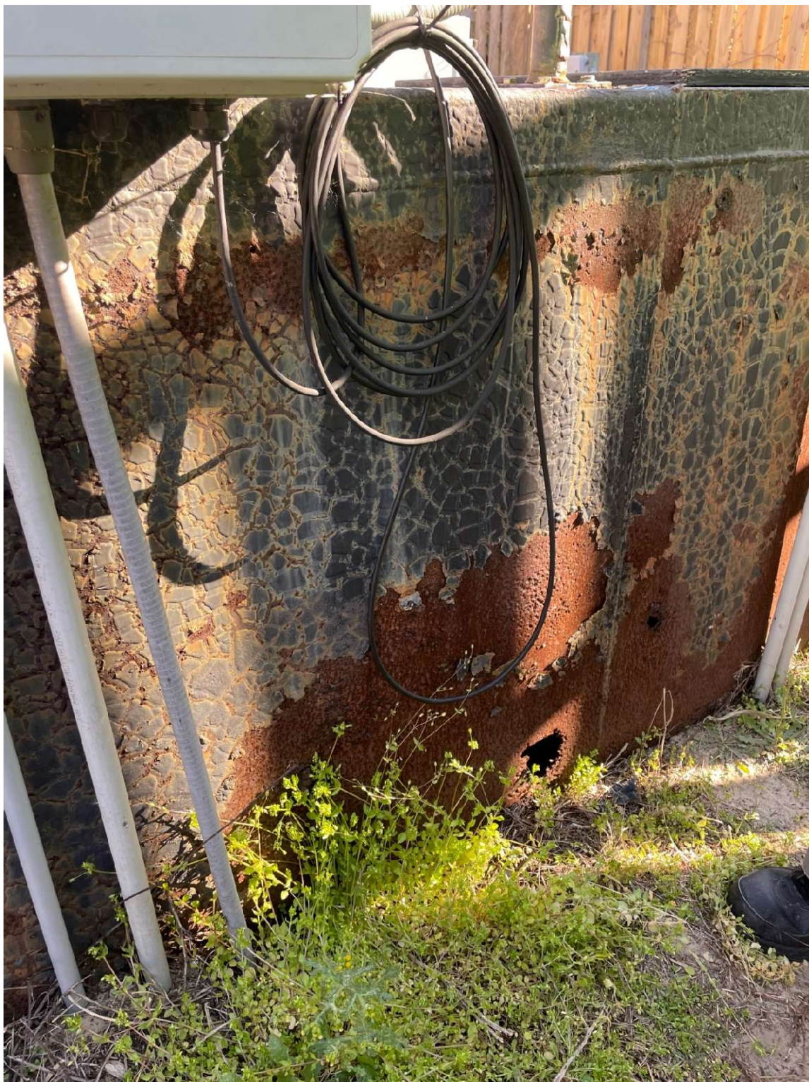
Back end of WWTP
