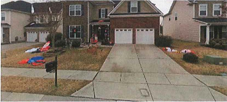
9702 Loughlin Ln Building
