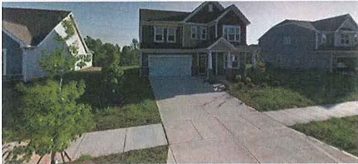
14726 Baytown Court Building
