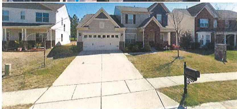
15132 Taylor Ridge Ln Building
