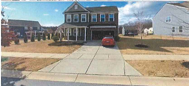
14213 Brancion Hills Ct Building
