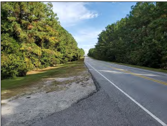
Looking east along US Hwy 101, subject on left
