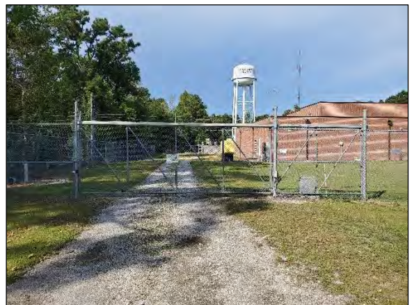
Looking north through west entrance to parcel
