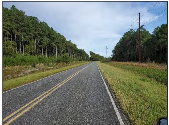
Looking east along Old Bridge Rd, subject on right
