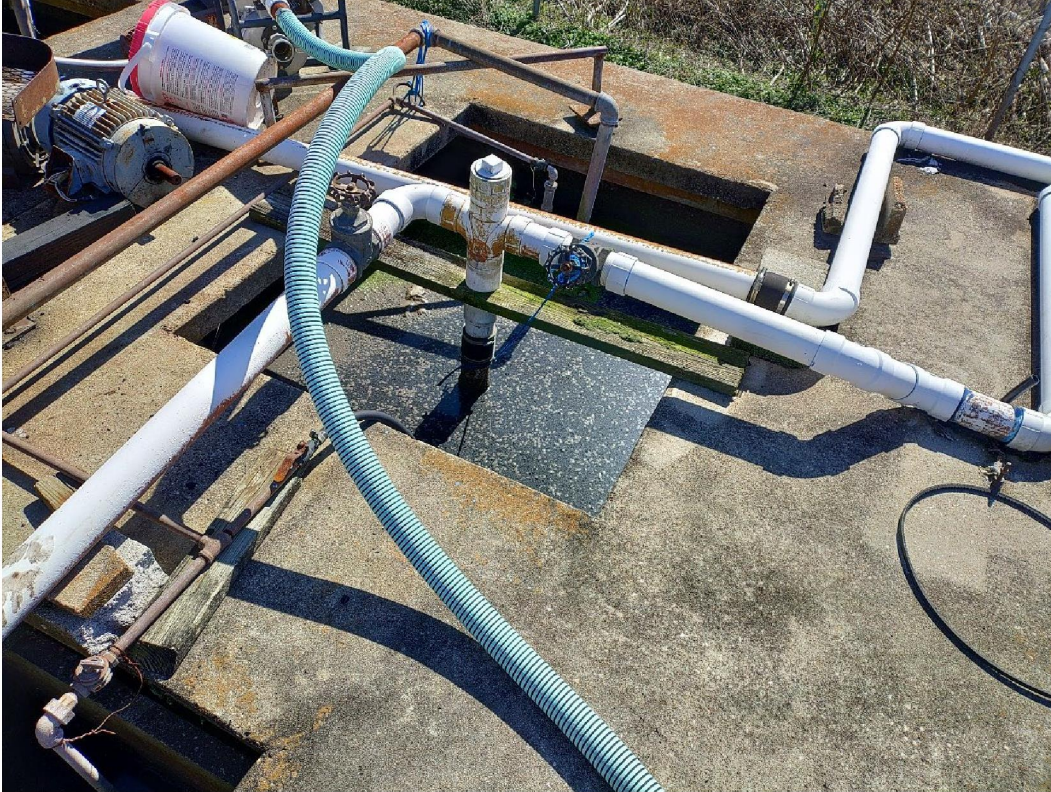
Figure 12. Clarifier tank (February 21, 2024).
