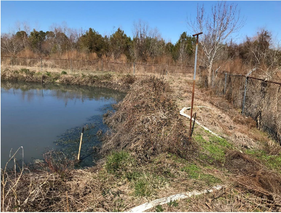
Figure 9. Storage structure with observed rack line along top of berm and past indication of overflow (February 21, 2024).
