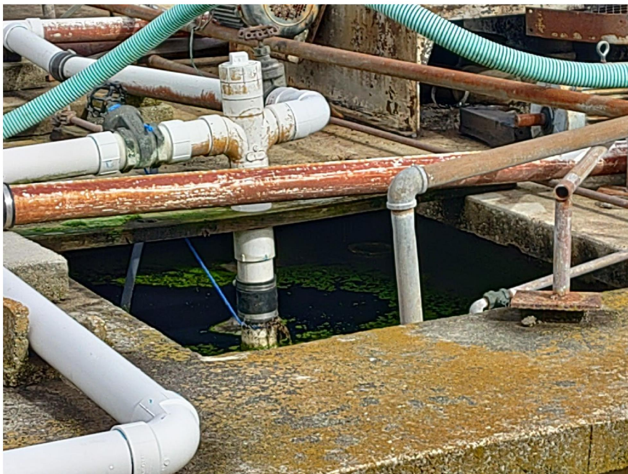
Figure 5. Clarifier tank (February 13, 2024).
