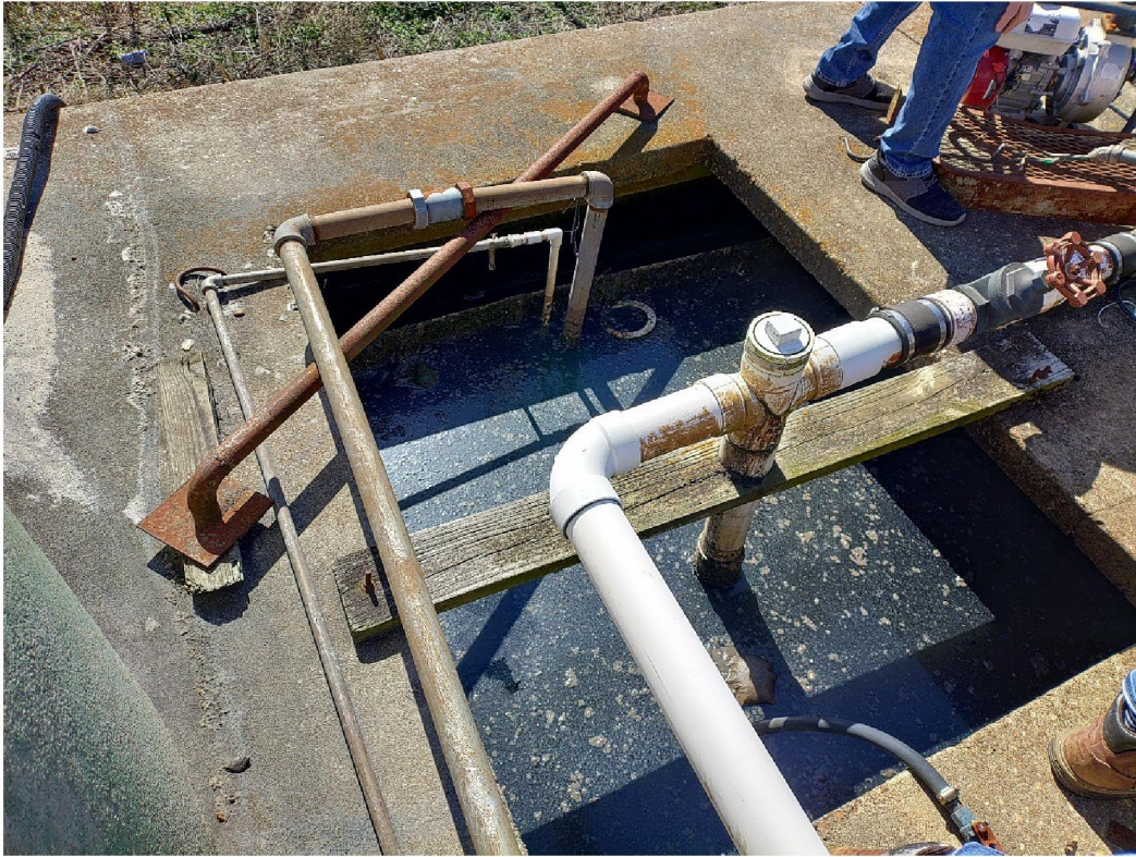
Figure 13. Clarifier tank (February 21, 2024).
