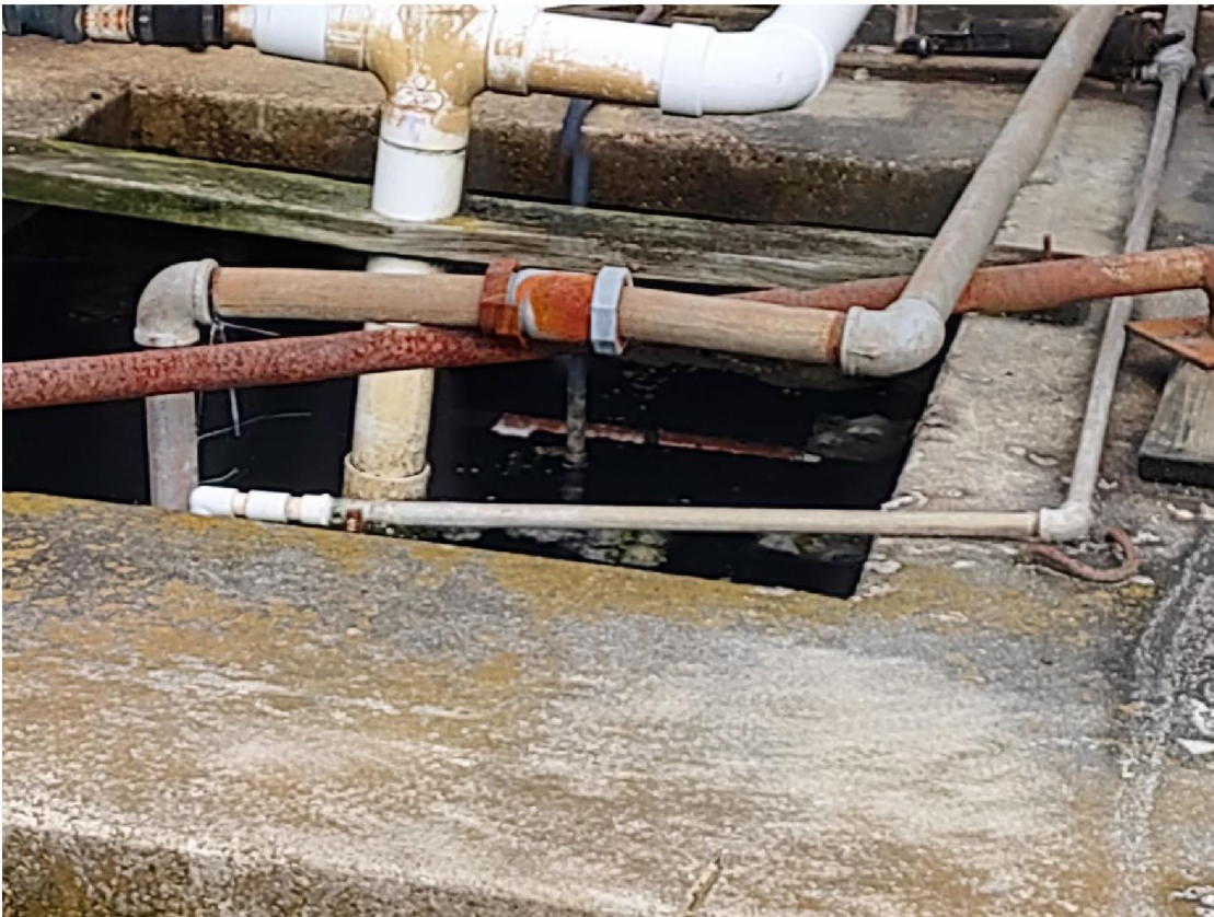
Figure 4. Clarifier tank (February 13, 2024).
