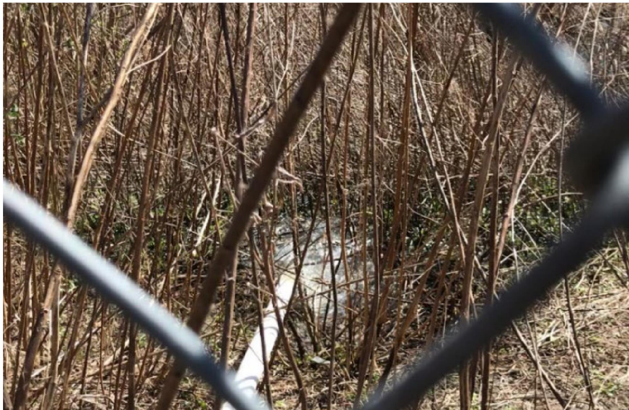
Figure 7. Unpermitted discharge, discharging wastewater (February 21, 2024)
