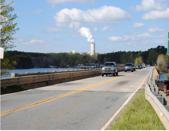
Resource CT1571, Bridge #138
