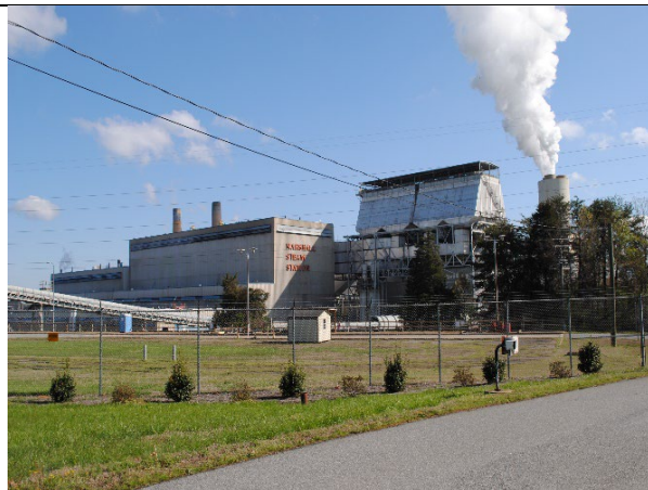
Resource CT1303, Marshall Steam Station
