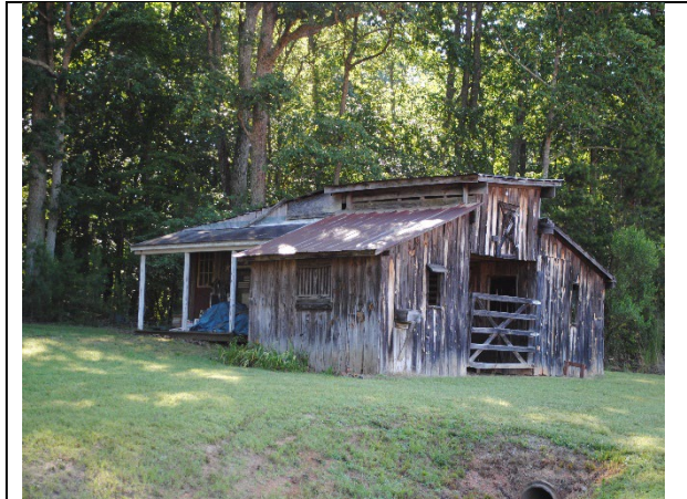
Resource MP-15, Barn on Raccoon Track Drive
