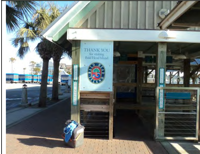
Side View Main Building
