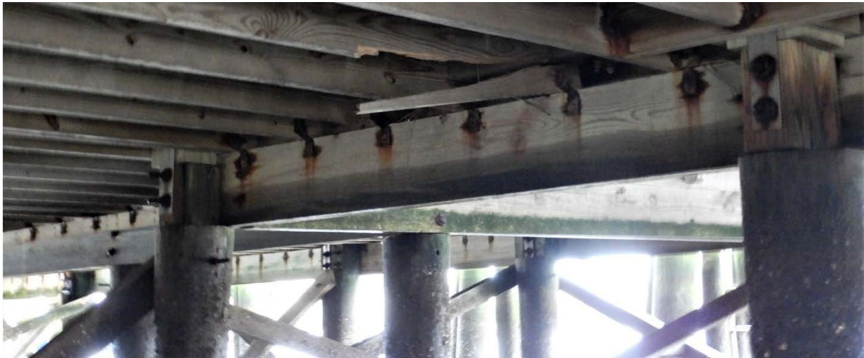
FIGURE 2-4: DPM B-GATE CONTRACTOR LANDING UNDER DECK FRAMING
