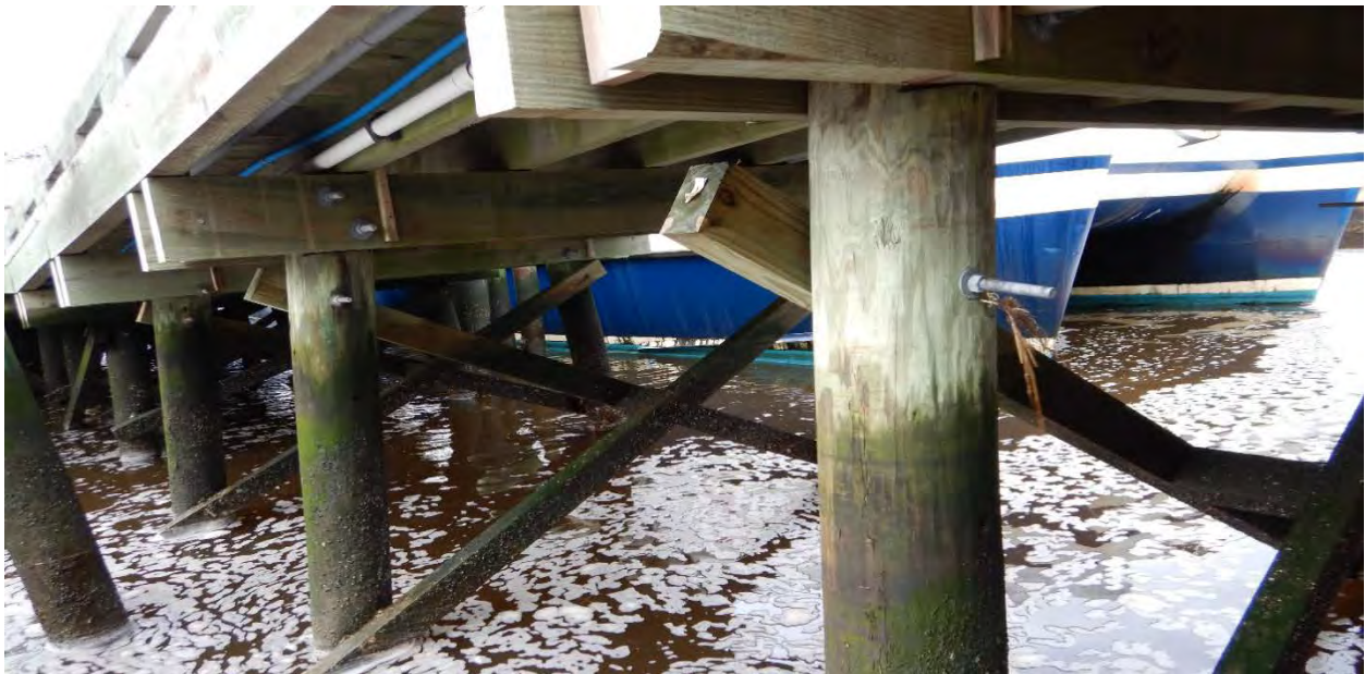
FIGURE 2-6: DPM MAINTENANCE FIXED PIER TIMBER PILE BENTS
