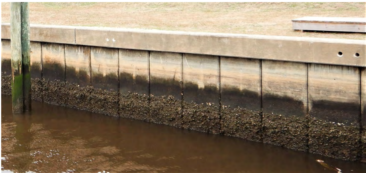
FIGURE 2-12: TYPICAL BULKHEAD WALL ELEVATION AT LOW TIDE
