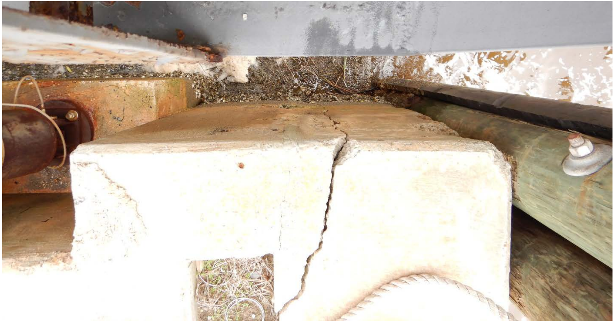
FIGURE 2-19: DPM BARGE RAMP TENSION CRACK IN CONCRETE SUBSTRUCTURE
