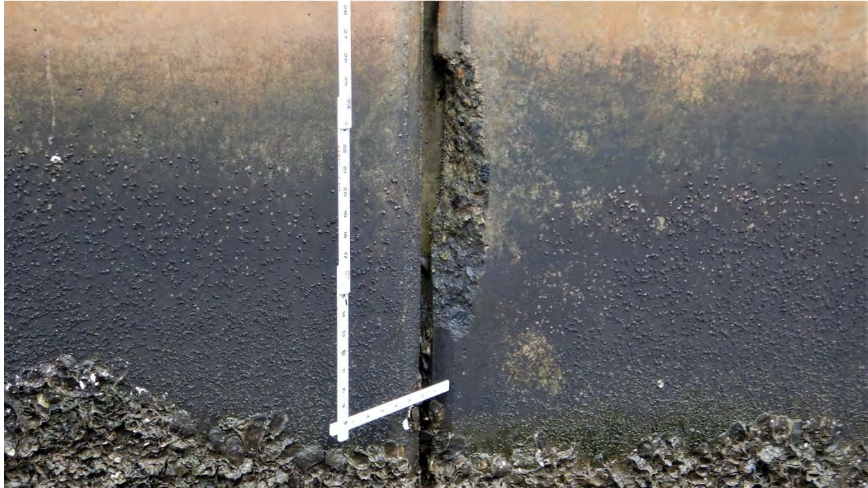
FIGURE 2-13: TYPICAL CONCRETE SHEET PILE SPALL
