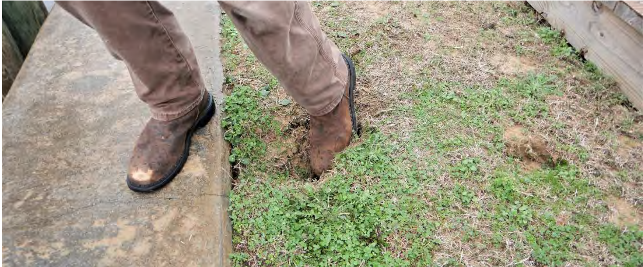
FIGURE 2-15: TYPICAL SINKHOLES BEHIND WALL
