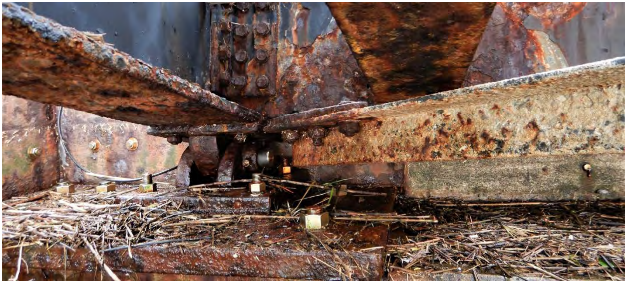
FIGURE 2-21: BHI BARGE RAMP STEEL FRAMING MODERATE CORROSION
