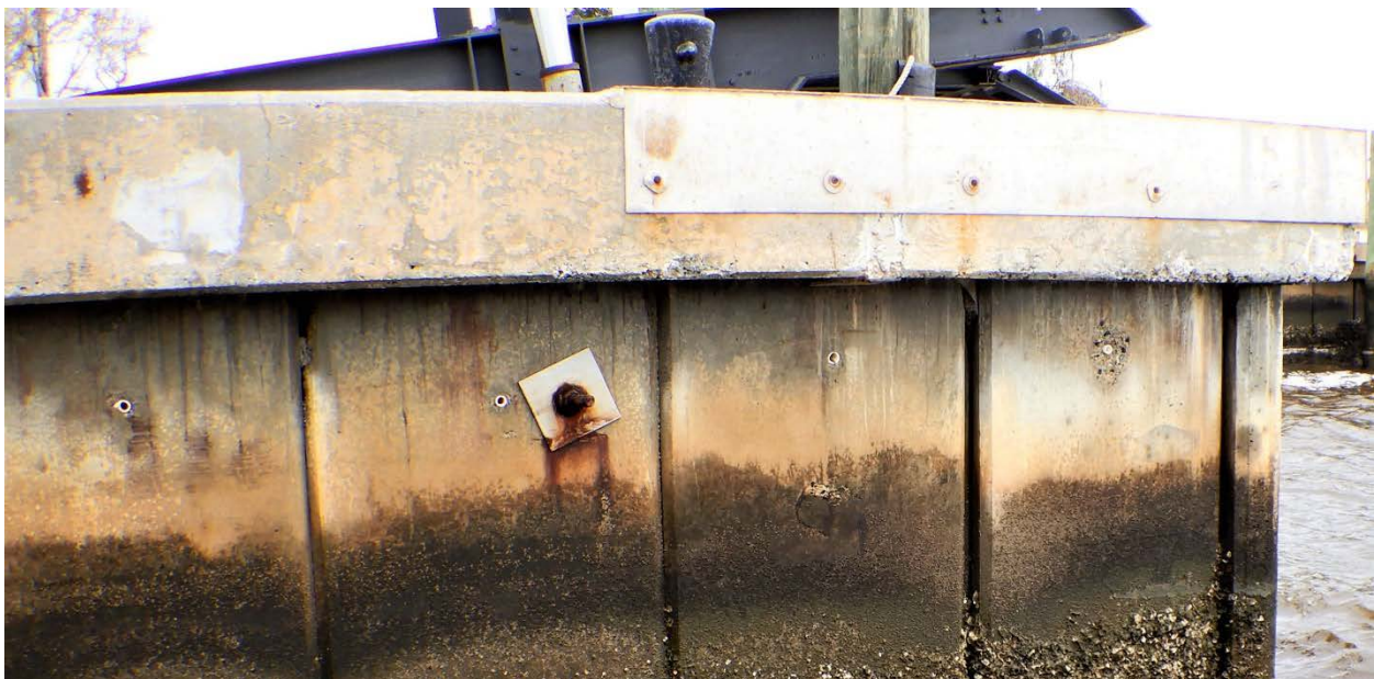
FIGURE 2-16: BULKHEAD REPAIR SECTION ELEVATION VIEW (LOOKING NORTH)
