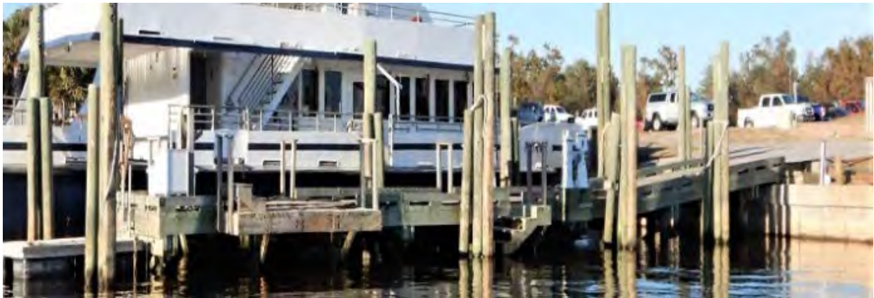
FIGURE 2-6: DPM MAINTENANCE FIXED PIER TIMBER PILE BENTS
