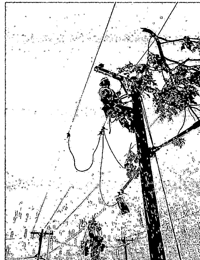
LINEMAN IN RAIN IN AREAS INACCESSIBLE BY BUCKET TRUCK, LINEMEN HAVE TO CLIMB POLES TO MAKE REPAIR
