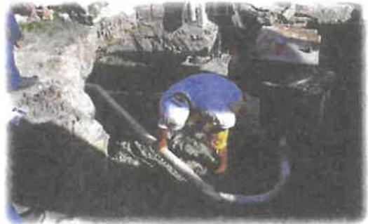
Interconnection process, of gravity and vacuum lines.
