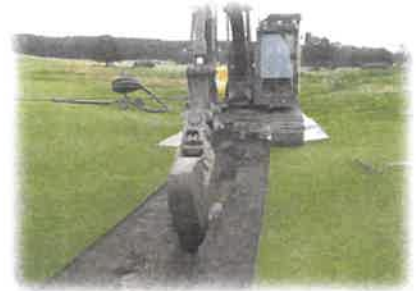
Typical excavation on golf course
