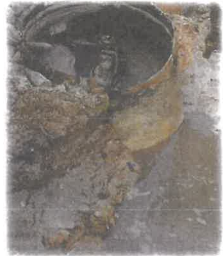
Airvac collector tank in poor condition, with serious leaks of sewage into the subsoil and water table.
