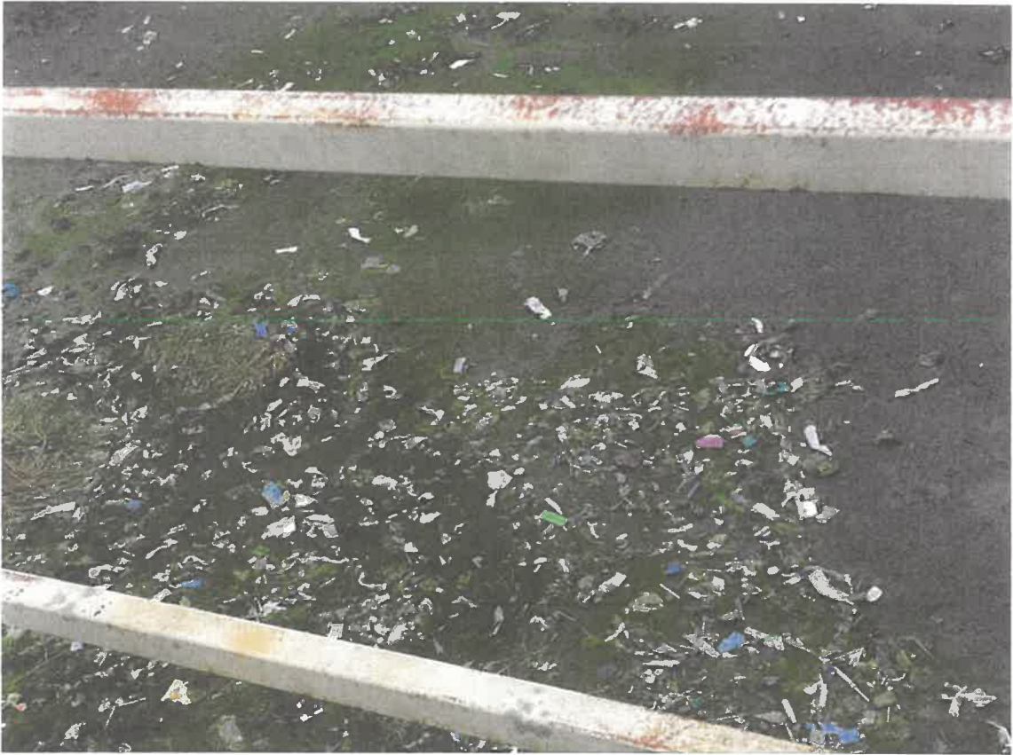
Photos: from August 4, 2020— Eagle Creek WWTP
