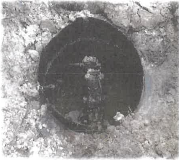
Airvac collector tank in poor condition, with serious leaks of sewage into the subsoil and water table.
