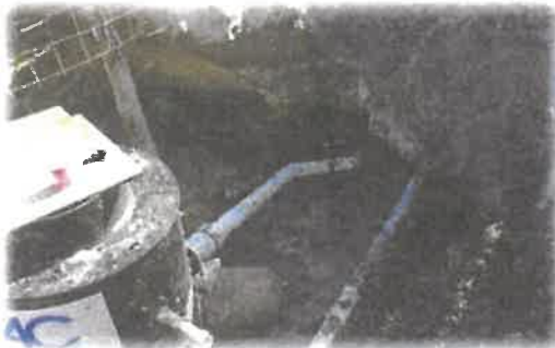
Interconnection process, of gravity and vacuum lines.
