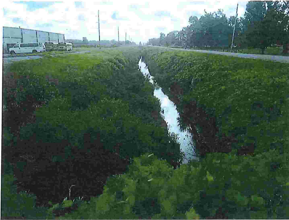
Photo 3: Looking east from intersection of Terra Ceia Road and Christian School Road at large canal that intercepts small canals. All project drainage exits to this tributary.
