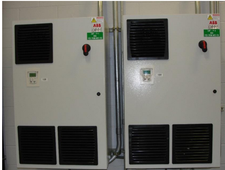
Figure 6. Primary Chilled Water Pump Variable Frequency Drives
