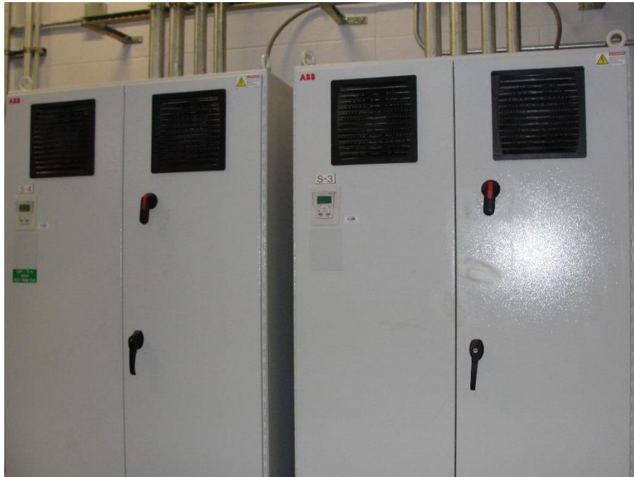
Figure 8. Secondary Chilled Water Pump Variable Frequency Drives
