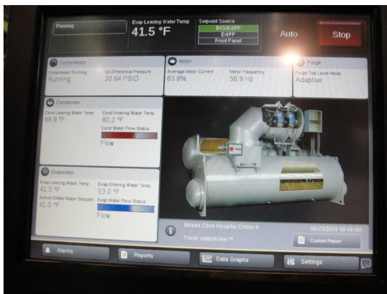
Figure 3. Installed Trane Chiller Control Panel
