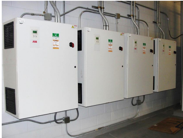
Figure 4. Cooling Tower Fan Variable Frequency Drives
