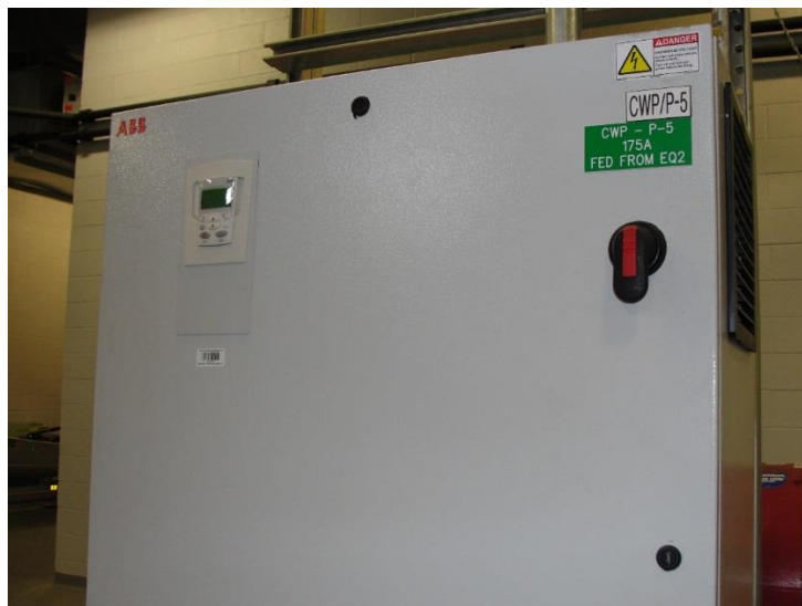
Figure 10. Condenser Water Pump Variable Frequency Drive
