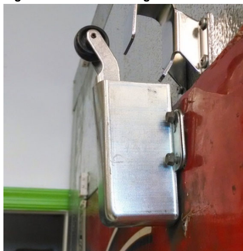
Figure 6-7. Malfunctioning walk-in door closer
