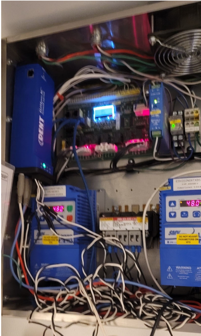
Figure 6-8: Dent Elite Power Meter Installed on VSD Kitchen exhaust fan
