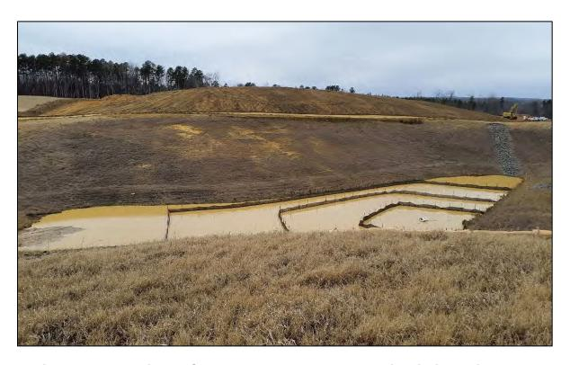
Figure 5.1-5: Drainage Control Pond and Mounded Fill within Project Area
