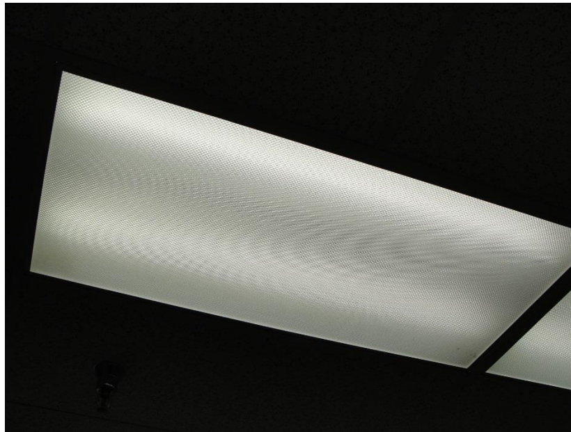
Figure 1. 2-Lamp, 2-Foot by 4-Foot T8 Troffer in Office
