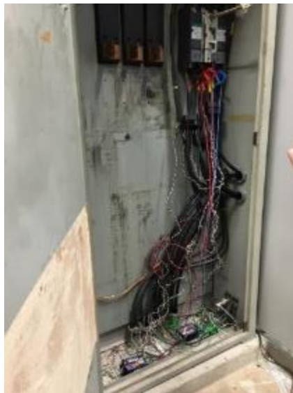
Figure 15. 250-hp VFD Air Compressor Meter Equipment Setup
