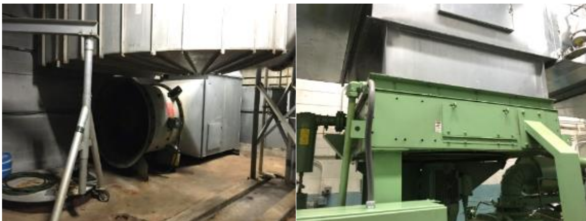
Figure 14. Compressed Air Heat Recovery System
