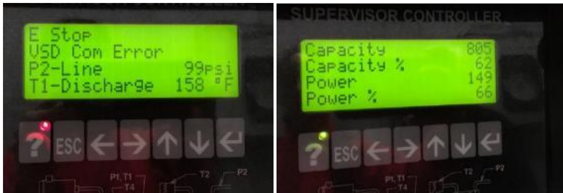
Figure 13. 250-hp VFD Air Compressor Control Screens
