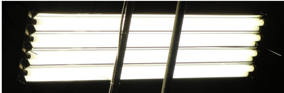
Figure 2. 4-Lamp, 4-Foot T8 Strip Fixture in Manufacturing Space
