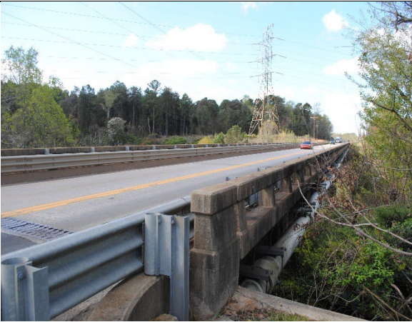
Resource CT1567, Bridge #117
