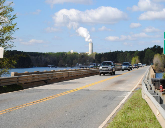
Resource CT1571, Bridge #138
