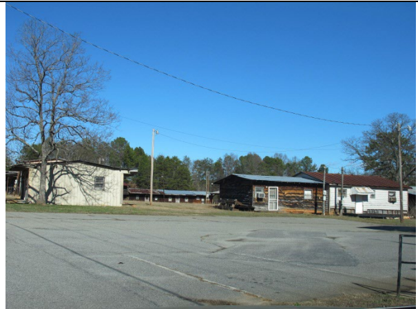
Resource CT0580, Mott's Grove Campground
