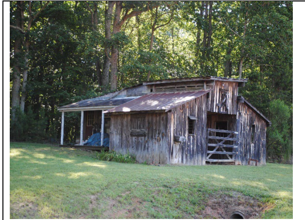
Resource MP-15, Barn on Raccoon Track Drive
