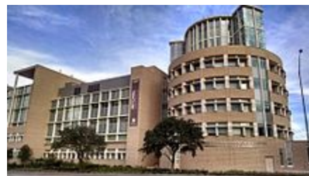
The Mitchell Physics Building on Texas A&M University's campus.
